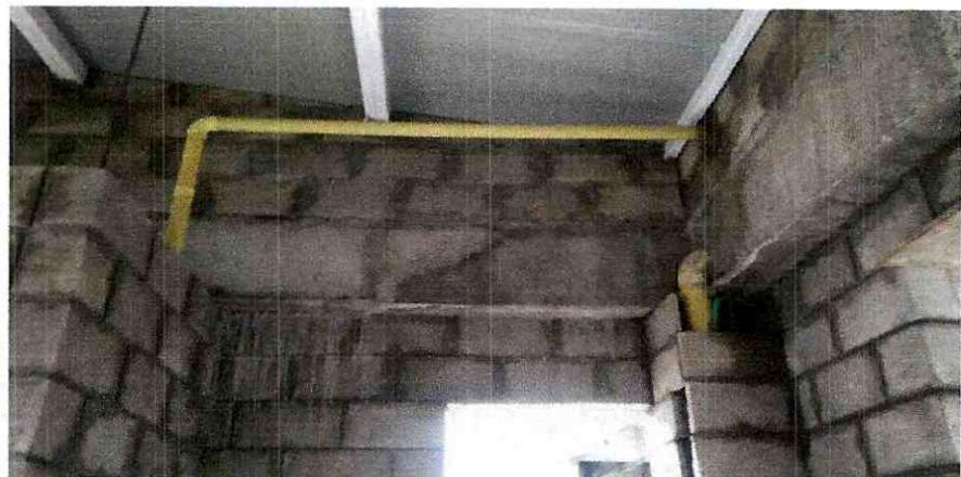
**SE SUBEN POR MUROS LA TUBERIA DE VENTILACION DE 2" Y SE SACA A LA PLACA**
